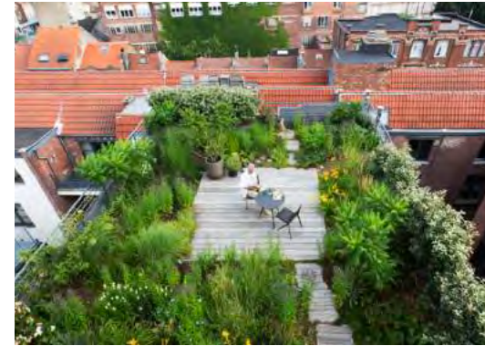
Roof gardens can provide amenity with a view
